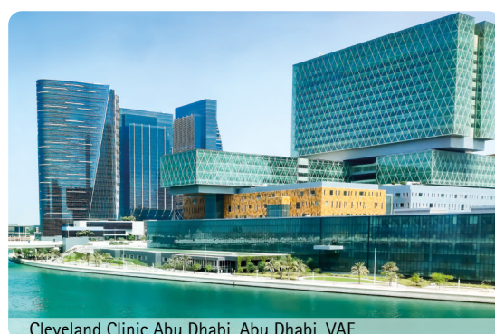
Cleveland Clinic Abu Dhabi, Abu Dhabi, VAE
