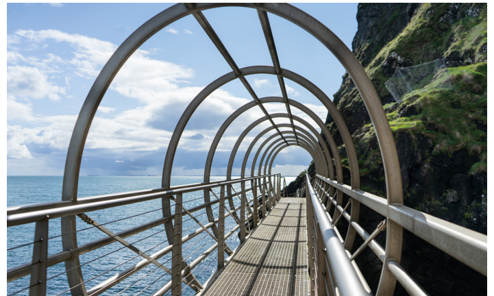
The Tubular Bridge
